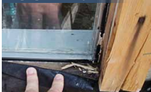
the result of improper flashing
