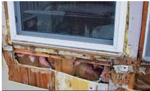
the result of improper flashing
