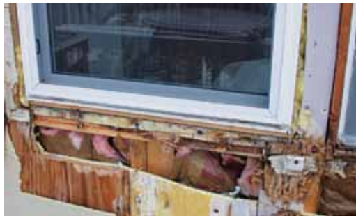
the result of improper flashing
